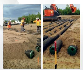
Covering the Advanced Enviro))Septic pipes with system sand
