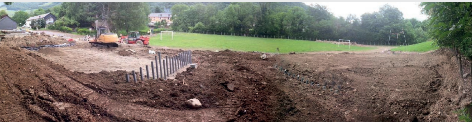
A panoramic view of the backfilled site
