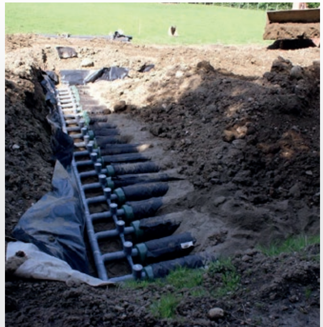
Covering the Advanced Enviro)Septic pipes
