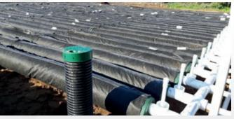
The injectors of the Low Pressure Repartition System
